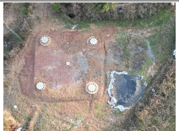
N11塔表土剥离、表土回覆、堆料铺垫塑料布
