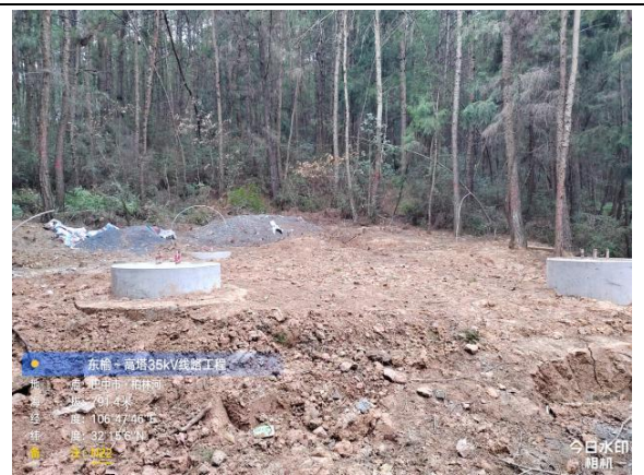
N22塔表土剥离、表土回覆、堆料铺垫塑料布
