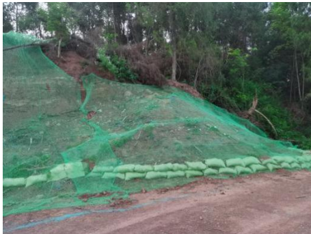
N008 塔基密目网苫盖，土袋拦挡
