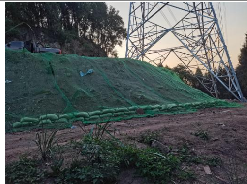
N033 塔基密目网苫盖、土袋拦挡
