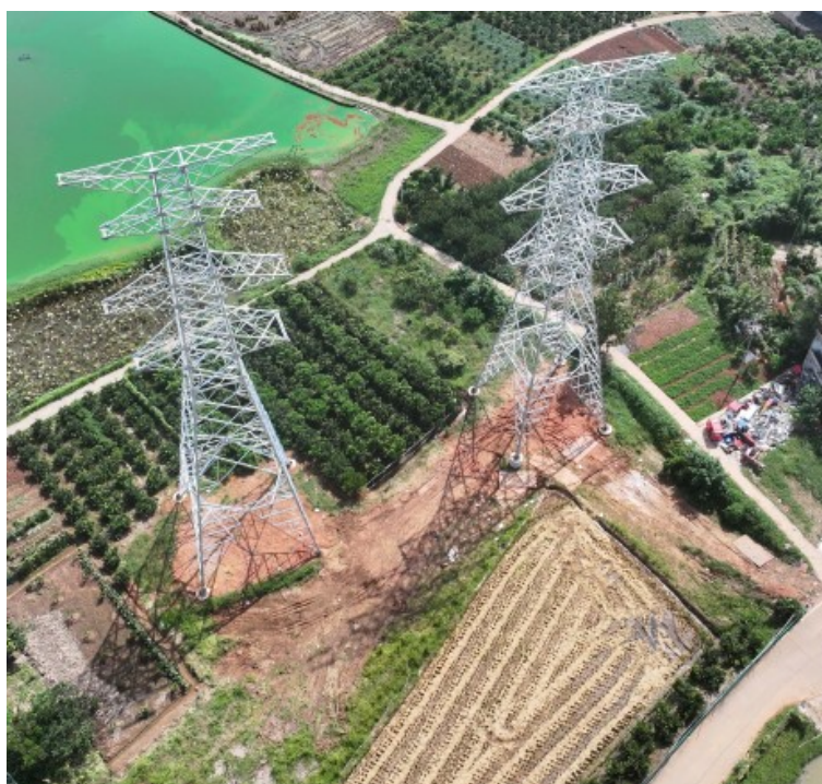
NB/NA12塔基裸露地表未苫盖
