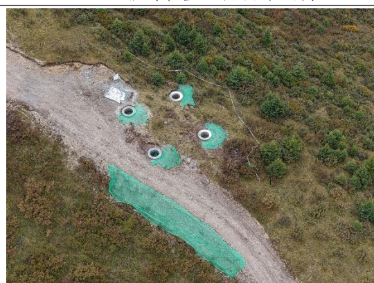
HR037 临时苫盖
