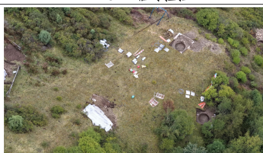
HL133G 临时苫盖
