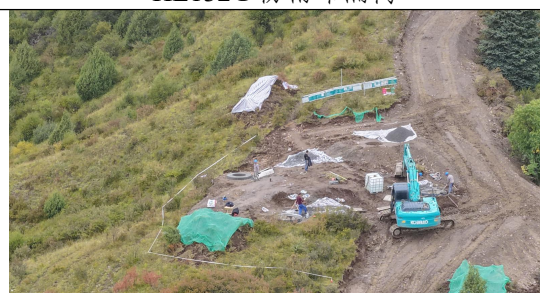
HR052 临时苫盖、防雨布隔离
