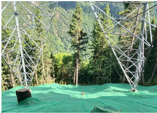
NAL58 临时苫盖
