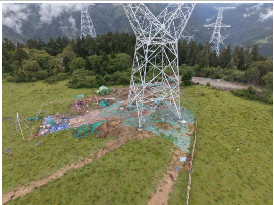
NAL5 临时苫盖
