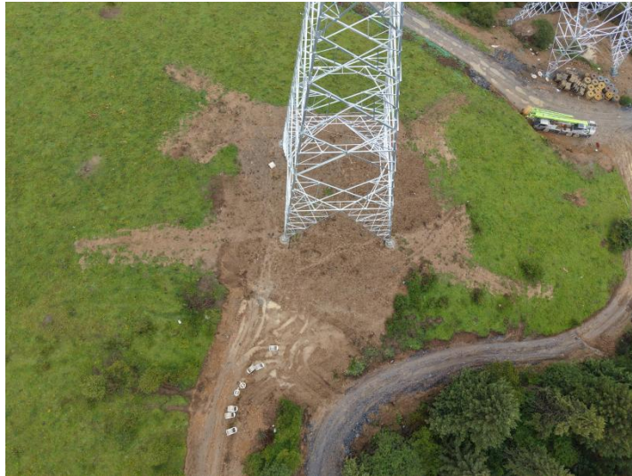
图3 N190塔基区无人机航拍
