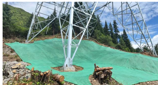
NAL57 临时苫盖
