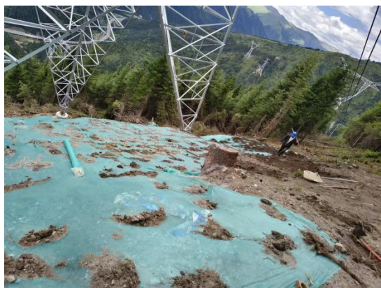
N171 临时苫盖
