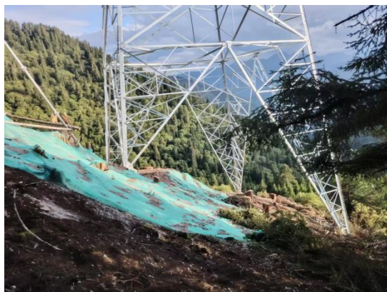
N174 临时苫盖
