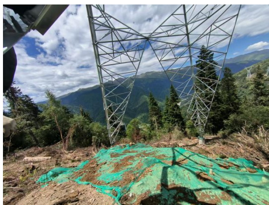
N170 临时苫盖
