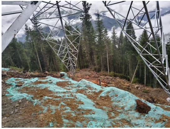
N185 临时苫盖
